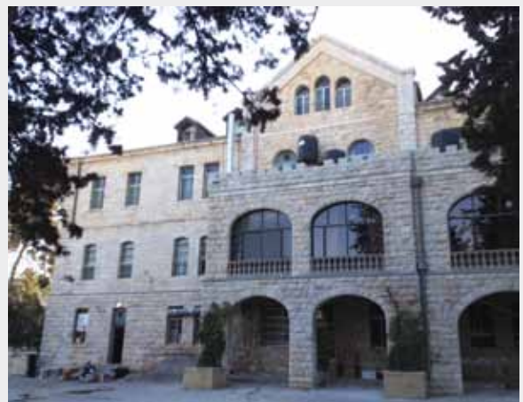
From the top: Before, during and after cleaning the administration building
